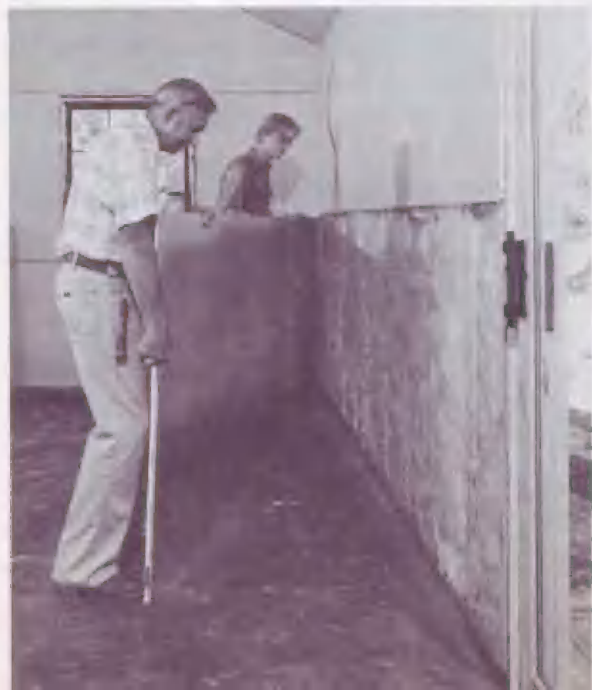
Gypsum board having one face covered with aluminum foil, shown here being installed horizontally, provides an interior wall with a vapor barrier.
